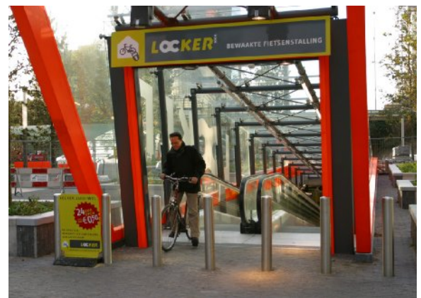
Locker station Amsterdam-Zuid
